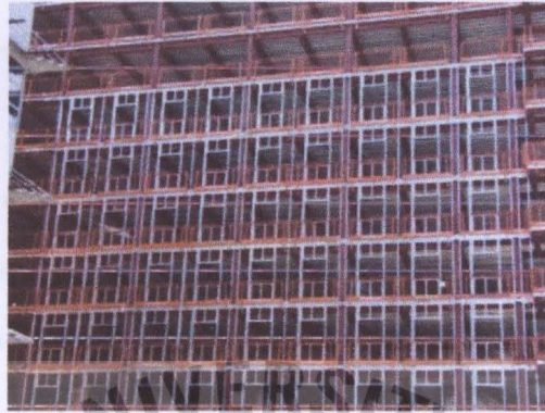
Figure 3.7 Typical light steel infill walls in a steel framed building
