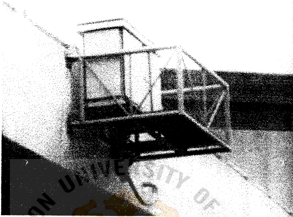
Figure 3.7. A Supply Pillar in a Basket.
