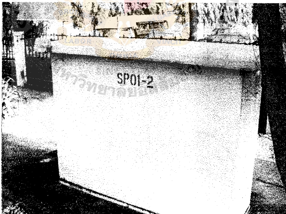
Figure 3.8. A Supply Pillar on Ground.
